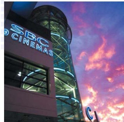
▲ Vue Cinema (formerly SBC) Hamilton, Scotland One of Solid State's many cinema installations, this project comprised a fully integrated fire alarm and voice alarm system
